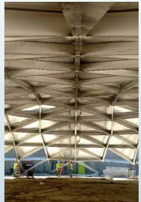
Construction of the Second Dickinson Reservoir
