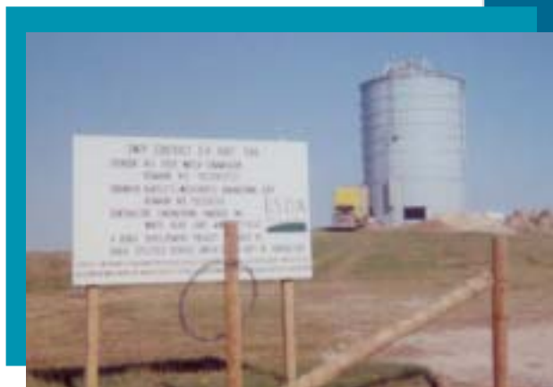
Burt Tank located near Mott, North Dakota.
